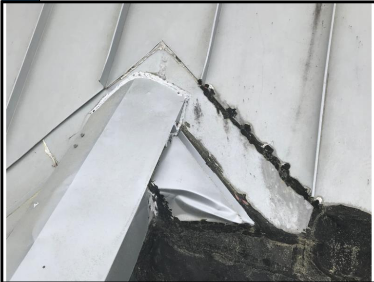
3 Asbestos results were negative for the white and black sealants.
