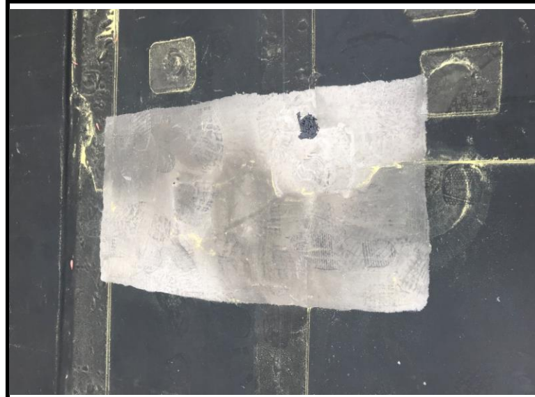
2 Asbestos results were negative for all roof patching material.
