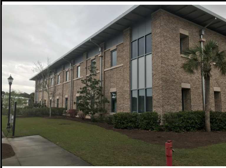
1 Typical exterior view of the Science and Technology Building on the USCB Bluffton Campus.
